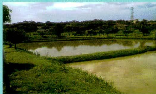
Plate 3: A well constructed fish pond
