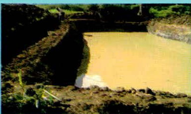
Plate 1: Construction of pond banks
