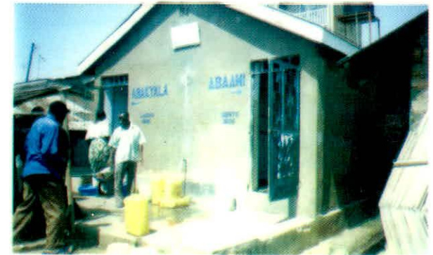
Toilet facility: One of the micro projects identified by the communities
