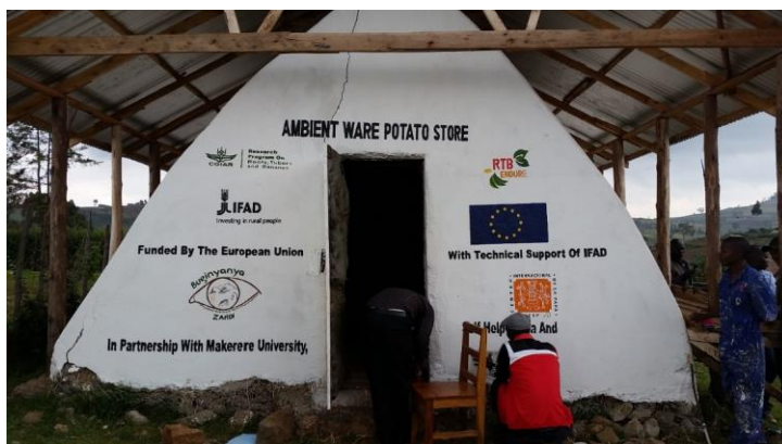
Figure 5: Front Exterior of a completed ambient ware potato store
