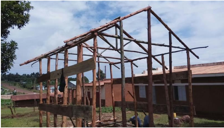
Figure 2: Framework of an improved wooden ware potato store
