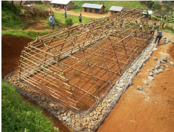
Figure 4: Framework of an ambient store before installing metallic re-enforcement bars
